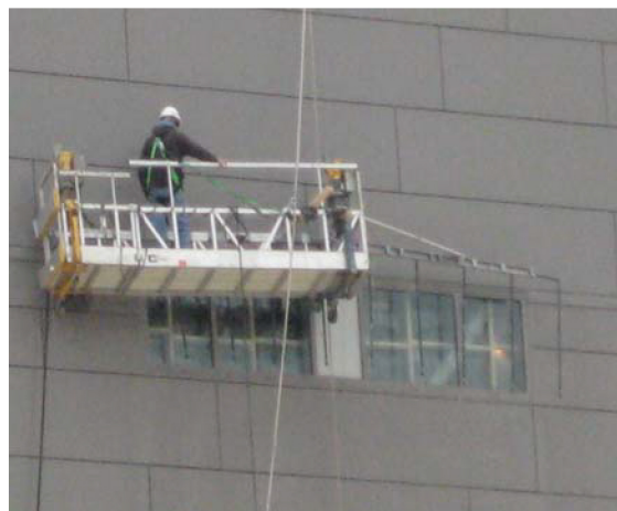
Photo 1: AAMA 502 Water Test
